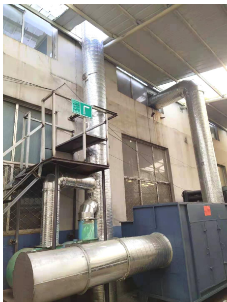
激光切割、焊接排气筒 P1
